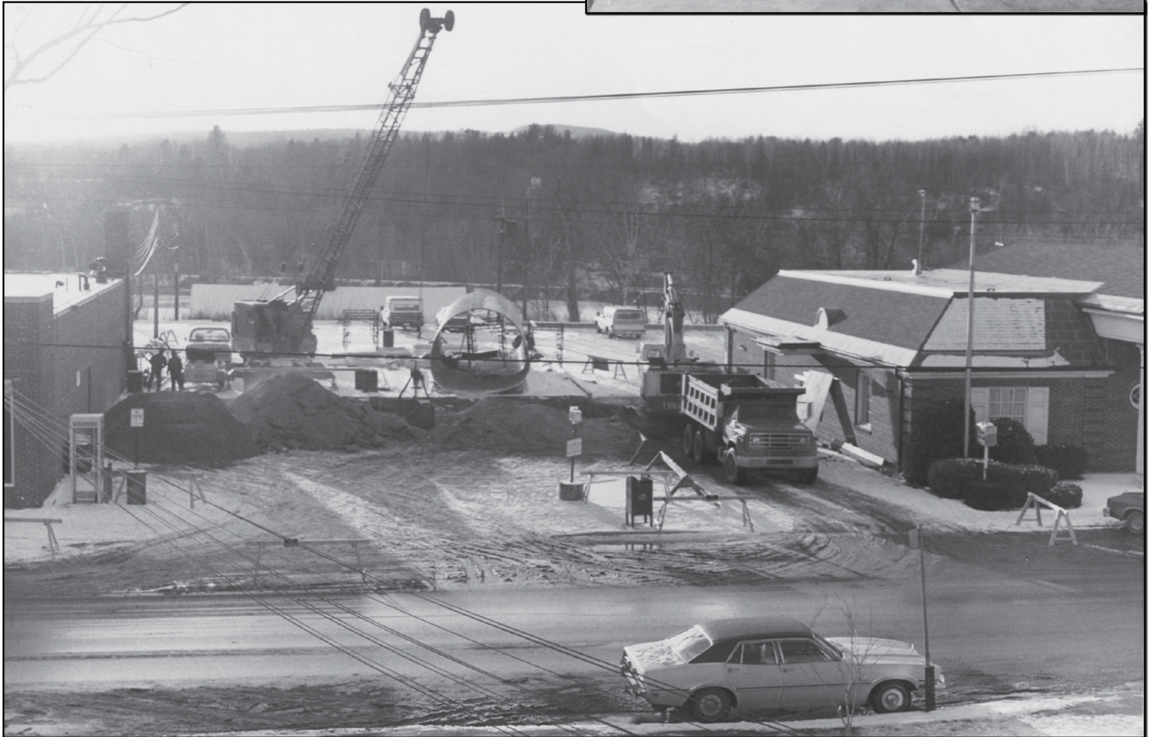
Installation of tunnel, a 78-foot long, 12-foot diameter steel culvert, and renovation of First National grocery store into new Loan and Operations Center, May 1980.
