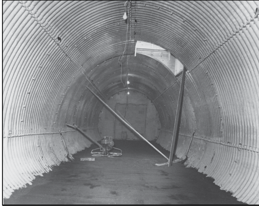
Installation of tunnel, a 78-foot long, 12-foot diameter steel culvert, and renovation of First National grocery store into new Loan and Operations Center, May 1980.
