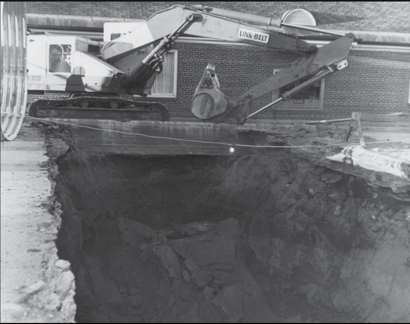
Installation of tunnel, a 78-foot long, 12-foot diameter steel culvert, and renovation of First National grocery store into new Loan and Operations Center, May 1980.
