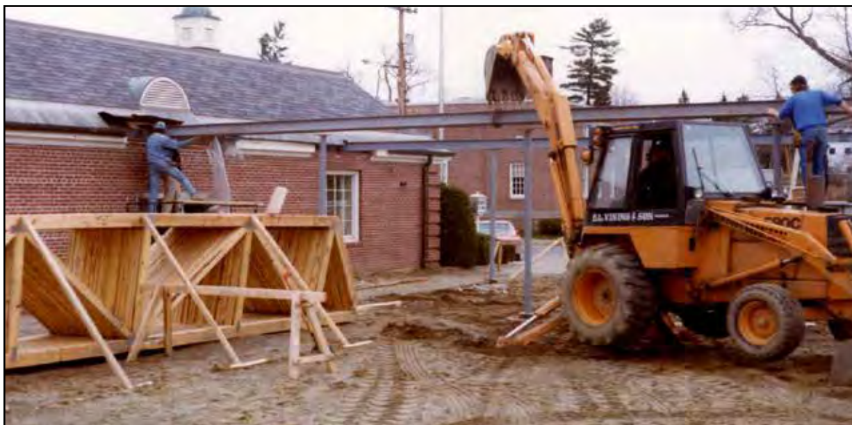
Finest Kind: Crews build a roof between the two buildings over the expanded drive-up. A mansard roof was added to the grocery store building, at right.
