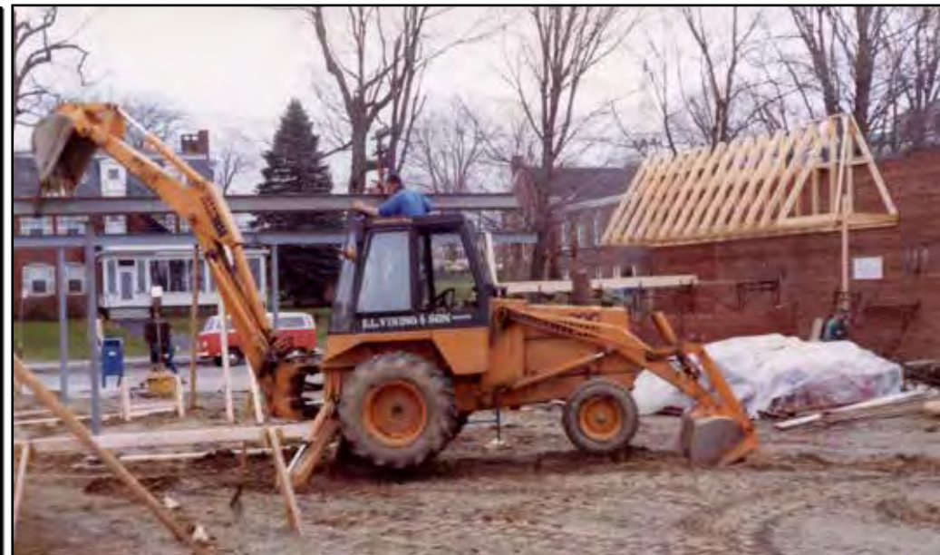
Finest Kind: Crews build a roof between the two buildings over the expanded drive-up. A mansard roof was added to the grocery store building, at right.
